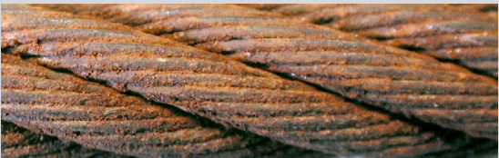
2. wires feel rough, general oxidation of the surface. Classification: 20 % of the discard maturity.
