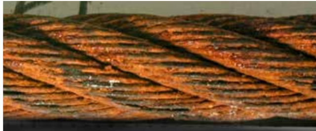
4. Surface heavily pitted and wires quite slack, gaps between wires – Discard immediately
